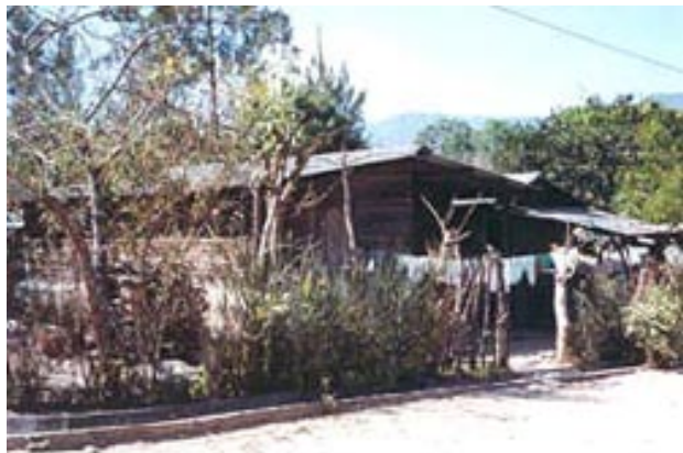
Poor Quality: The House in Pacux
